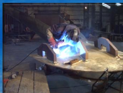
SMS Welding in Portugal.
